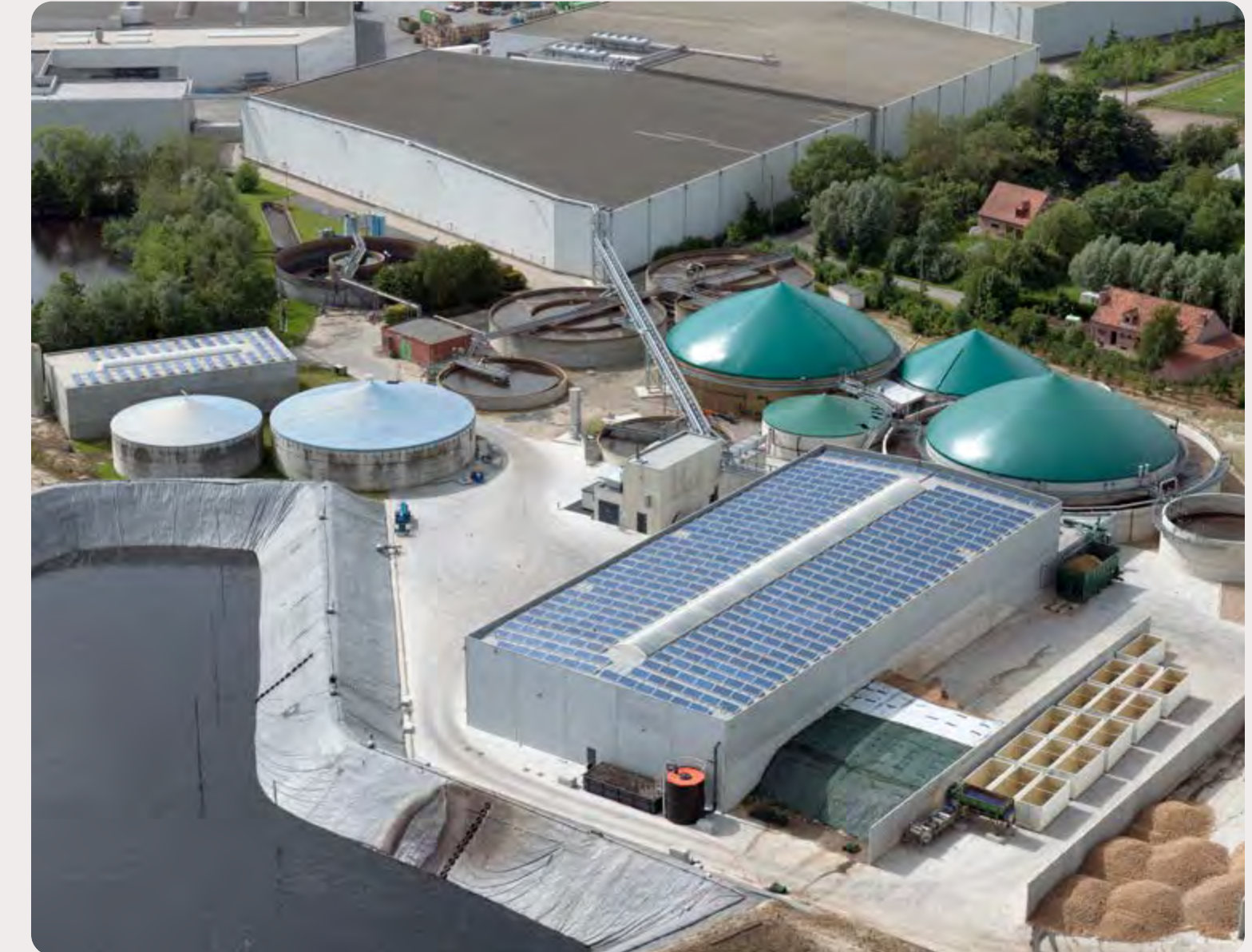
Green electricity and green steam generated at the biomethanisation plant in Ardooie (BE)
